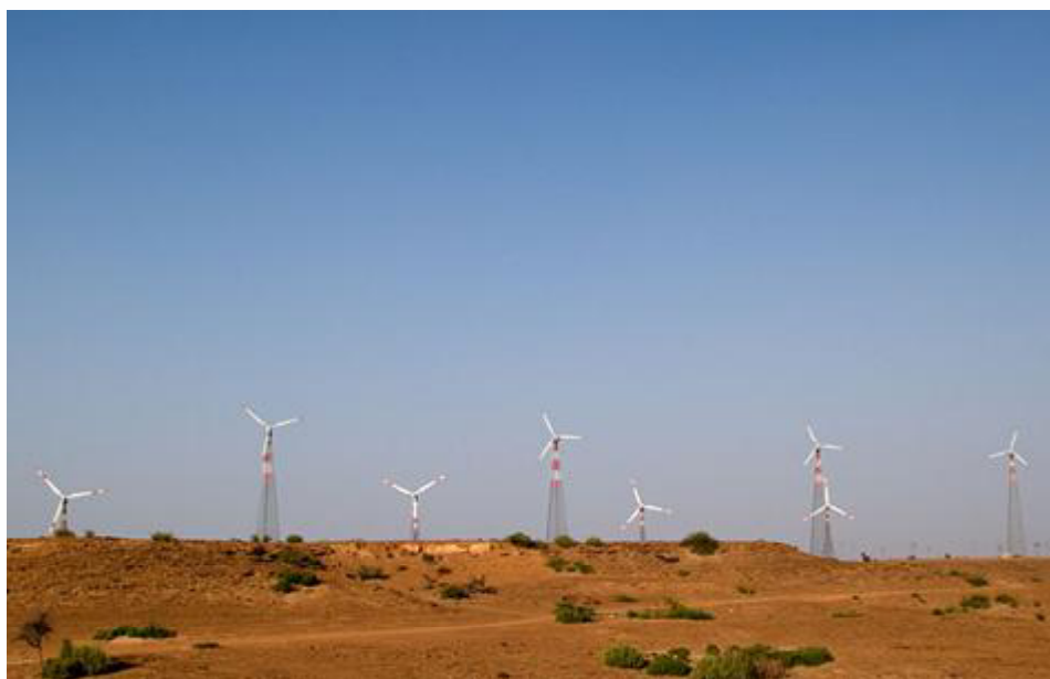
Fig. 7.10: Use of renewable energy as wind pump.
