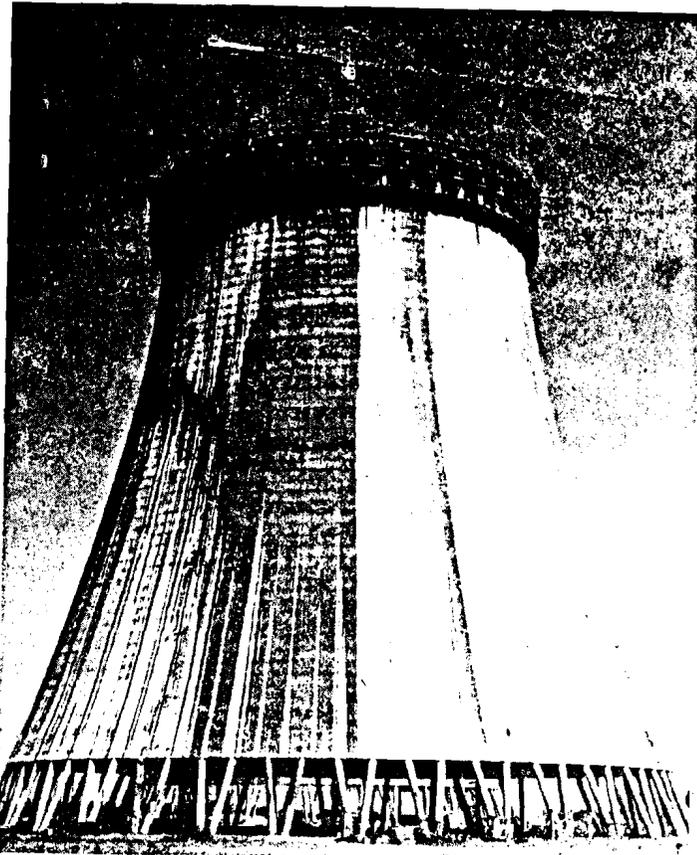
Figure 16.13 : Automatic Climbing Formwork for Cooling Towers
