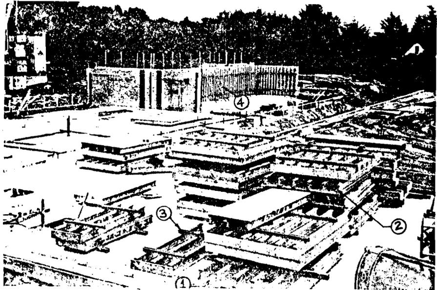
1. Plywood                      2. H-16 Beam                      3. Steel Walers                      4. Adjustable Props
