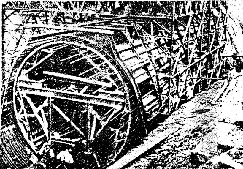
Figure 16.14 : Travelling Formwork
