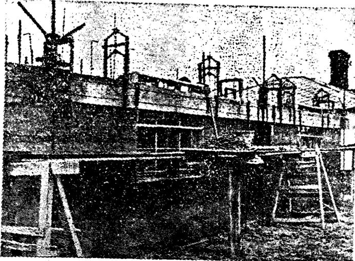
Figure 16.9 : Climbing Formwork
